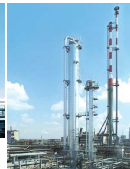
600 mtpd two-column distillation (grade AA Methanol) for BASF AG Ludwigshafen, Germany
